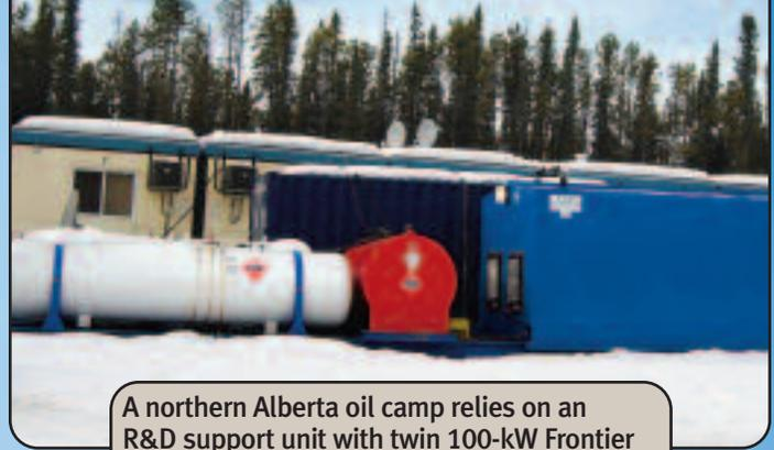
A northern Alberta oil camp relies on an R&D support unit with twin 100-kW Frontier gen-sets, enclosed in a blue doghouse.
