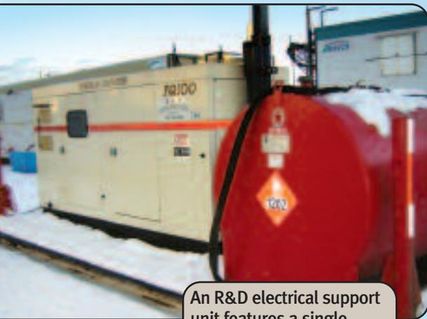
An R&D electrical support unit features a single 100-kW Frontier gen-set.
